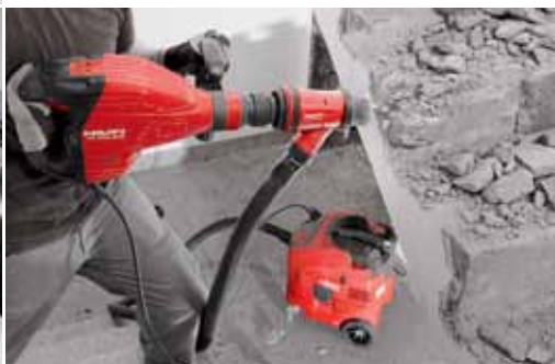
Removing screed and coatings on stairs virtually dustlessly.
